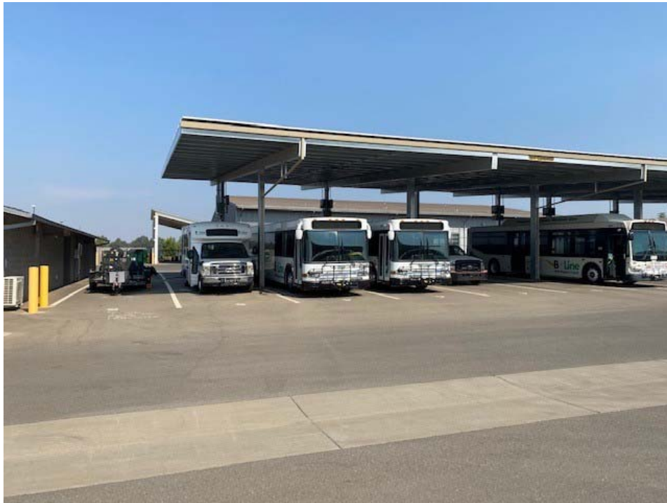
Northerly at bus solar canopy and expected charging head locations/area
