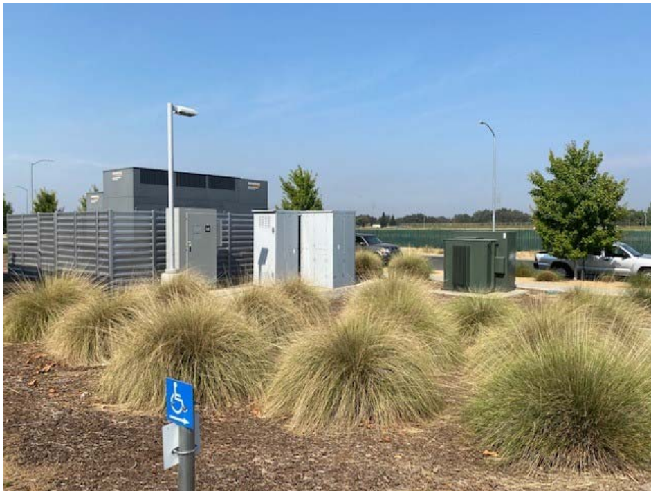
Existing switchgear at northeast area of campus property
