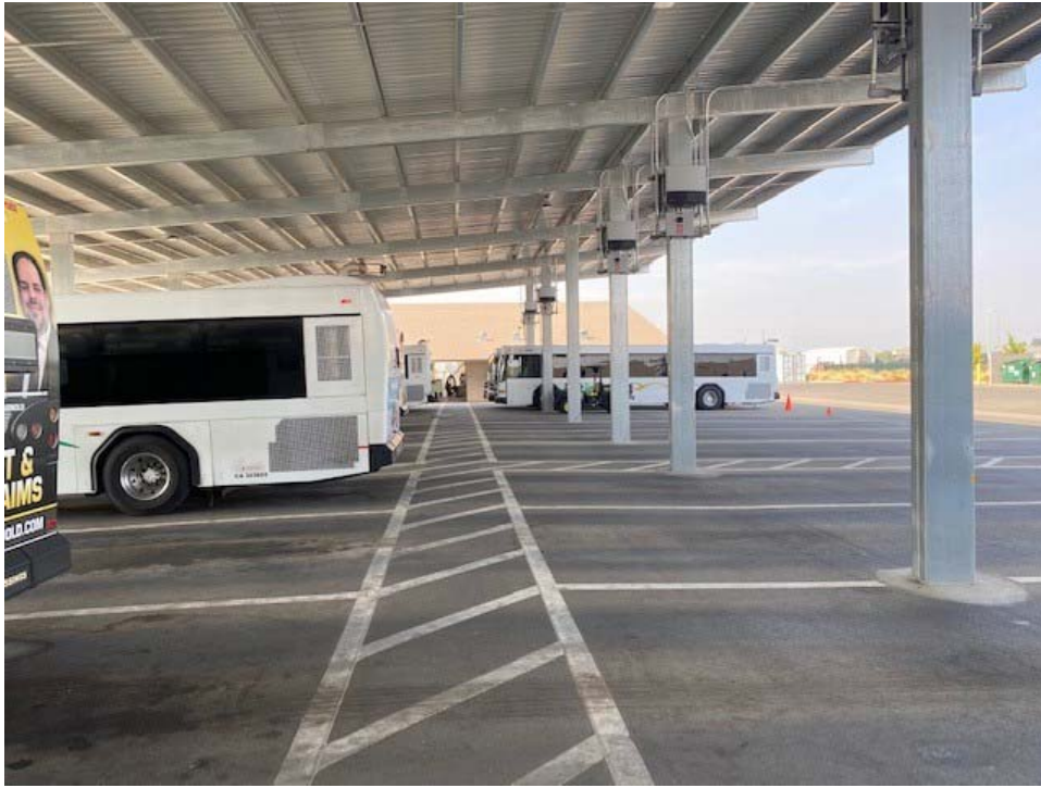
Westerly at bus solar canopy parking in direction of expected (future) charging head locations/area
