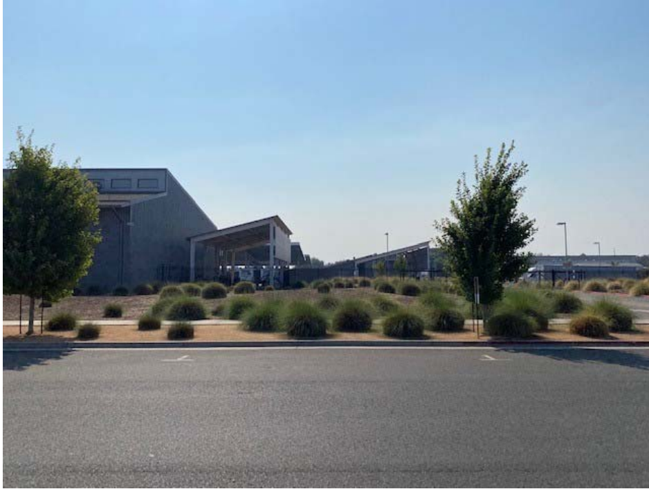
Southerly at possible new electrical service (location #1)
